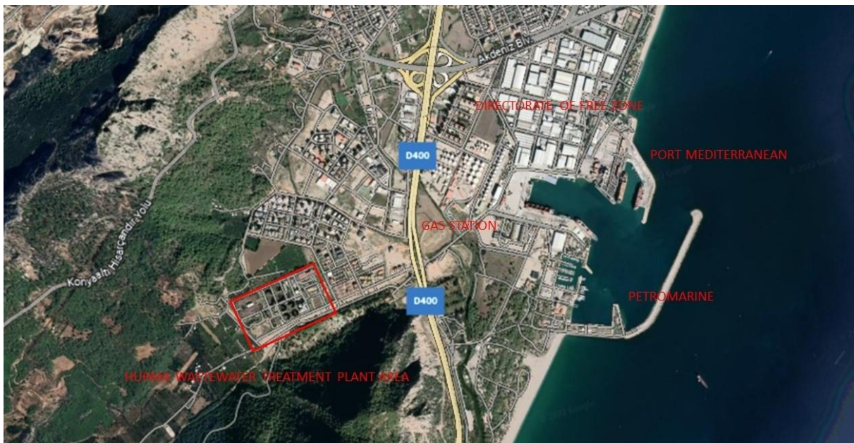
Figure 6. Surrounding of Hurma WWTP
