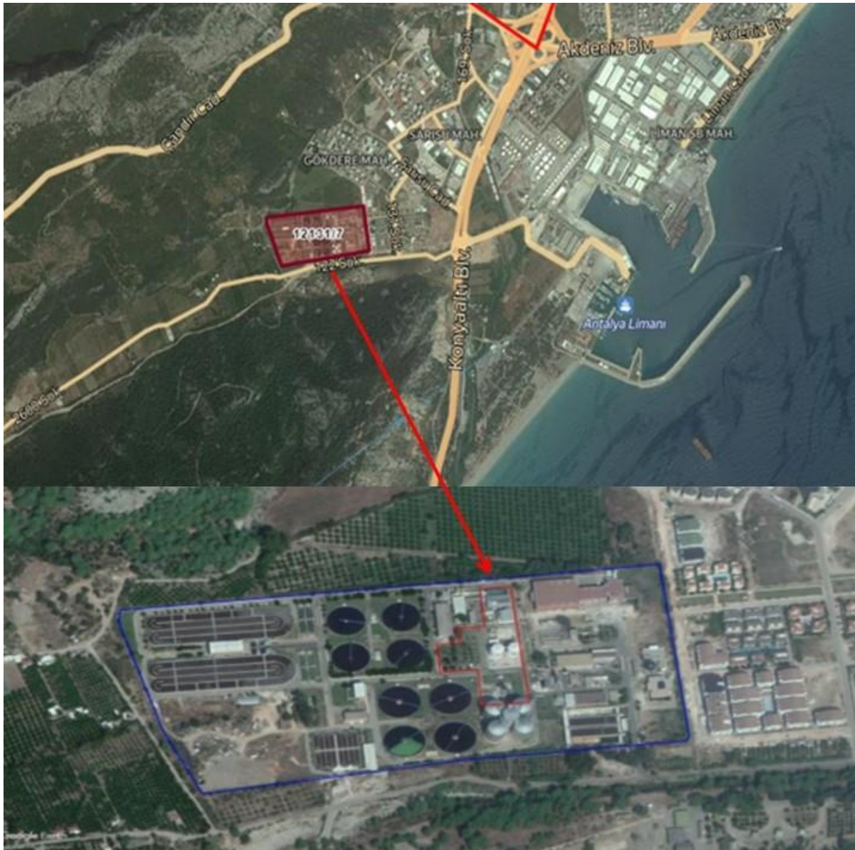
Figure 4. Aerial view of the existing Hurma WWTP (coordinates: 36°50'11.4"N 30°35'06.1"E)
